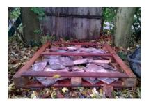
Fill the pallet with broken tiles or a similar heavy material.
